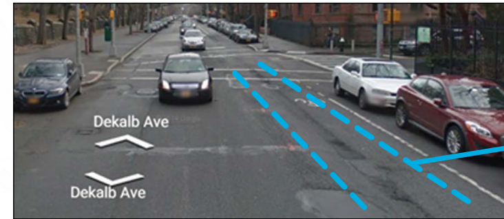
Dekalb Avenue in Brooklyn No protection in bike lane, bike lane paint is worn off, a lot of potholes
